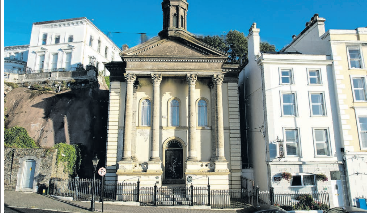
Pillars, a free-standing, three-bay, three-storey former Methodist church is guiding €500,000
